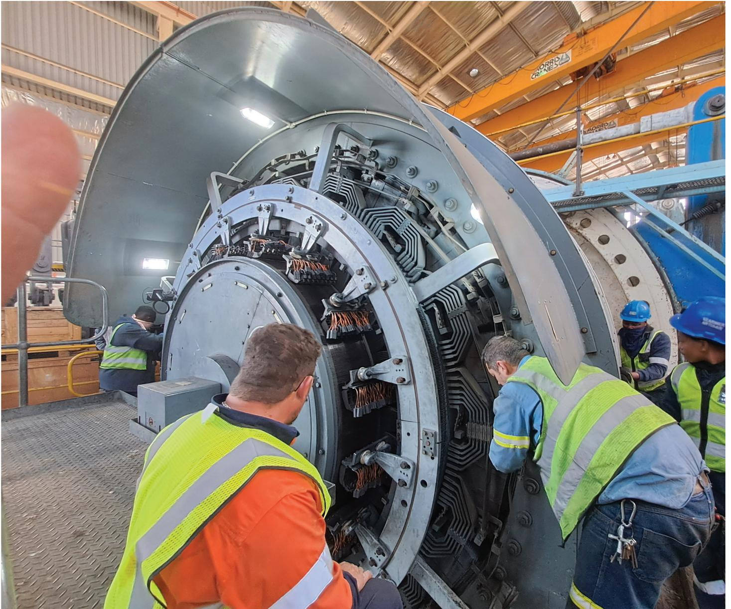
*Danie Gouws, M&C's Chief Field Service Technician (in orange shirt), assists the mine's technical personnel install the rock-winder motor into the man-winder position.*
