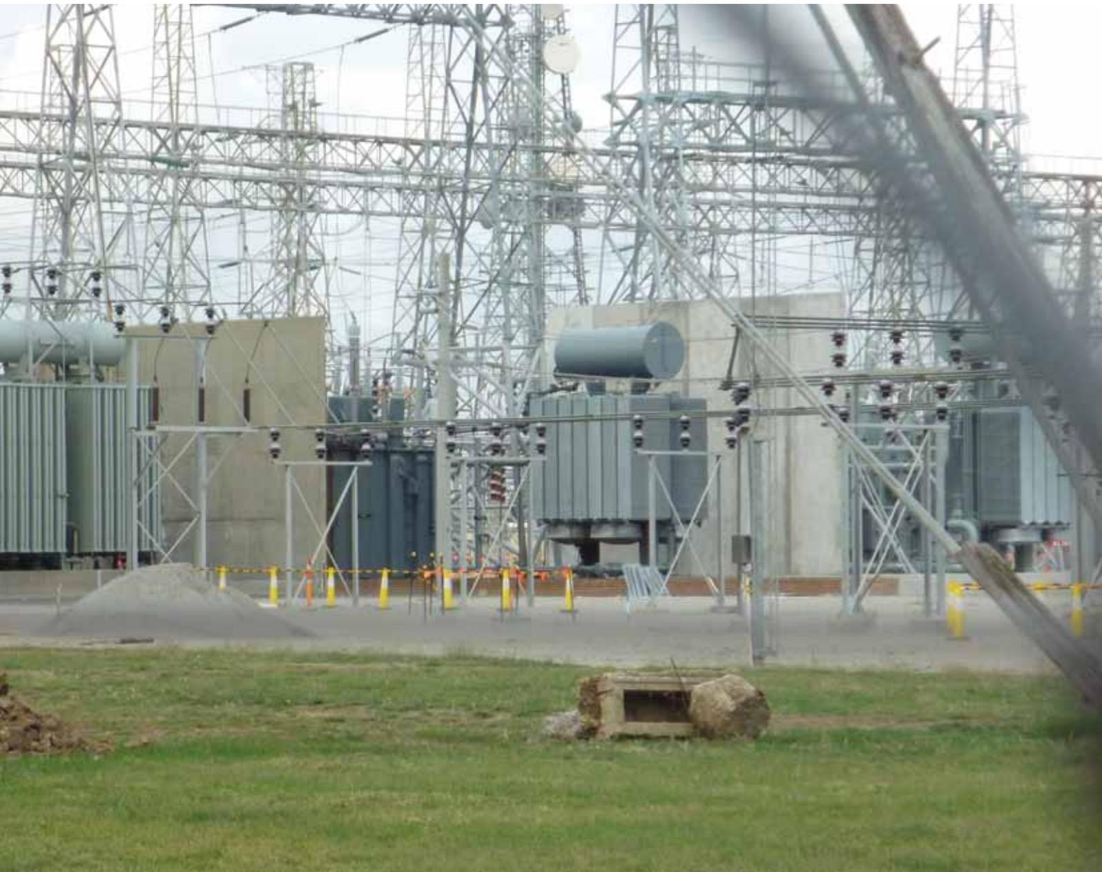
Circuit Breakers (OCBs) when a fault occurred. Both the circuit breaker feeding the fault and the incoming circuit breaker failed to trip. The upstream protection was slow in operating and the circuit breaker feeding the fault exploded, killing both of the electricians in the substation. In the ensuing accident investigation it was found
